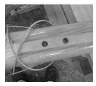
If you are retrofitting the track to your mast, you need to sand off the varnish where the batten will be epoxied to the mast.
