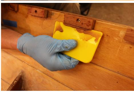
The spacer blocks are installed and the epoxy has cured.
