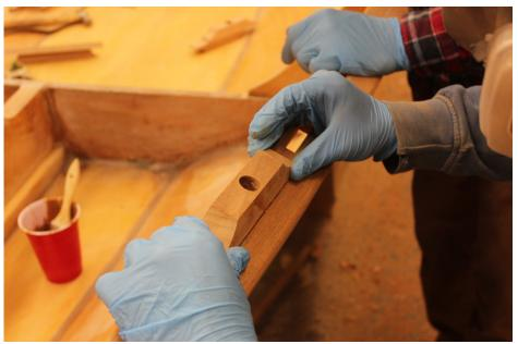
Spread epoxy on the oarlock risers and clamp them atop the rails.
