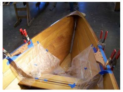
A hole for the mast must be created in the thwart, measuring 2-1/2" (63.5mm) square.
