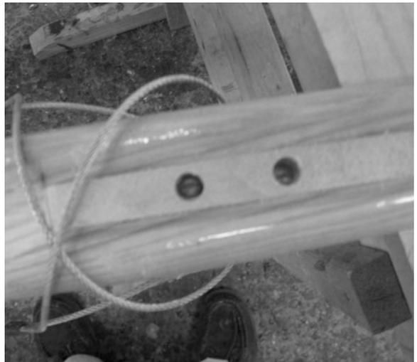
If you are retrofitting the track to your mast, you need to sand off the varnish where the batten will be epoxied to the mast.
